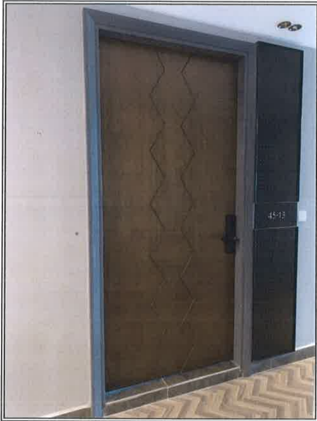
View of the entrance to the Property.
